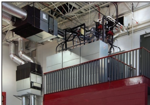
Eight rooftop HVAC units were replaced by a state-of-the-art mini-split heat and air cooling system with a geothermal loop and HRVs.
